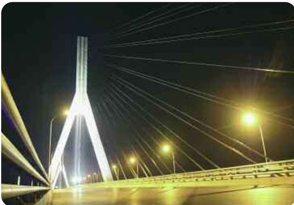
Donghai Bridge in Shanghai installed with Standby 250W HPS lamps
